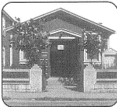
West Aliquippa Church Building on Erie Avenue
