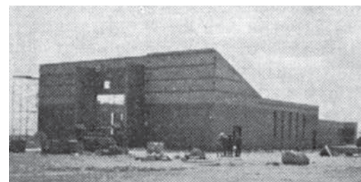
Auditorium building under construction ▶
