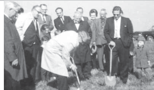
Groundbreaking at the World Operations Center ▶
